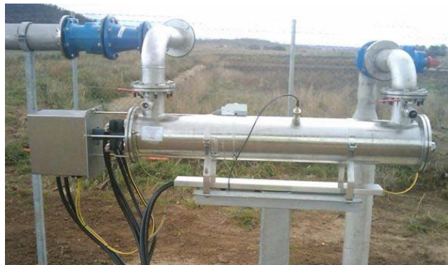
UVG X4-440-AW with automatic wiper at Berridale STP
