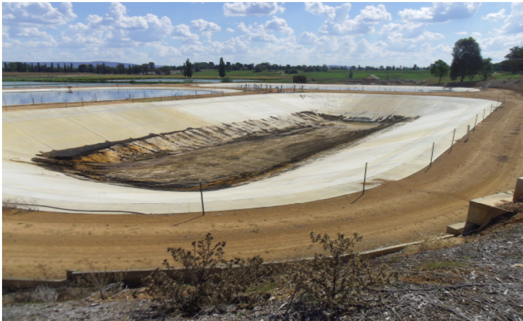
Figure 1: Emptied lagoon sand filter and underdrainage removed
