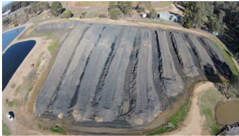
Figure 2: Windrows of Biosolids Stockpiled at the TWTP
