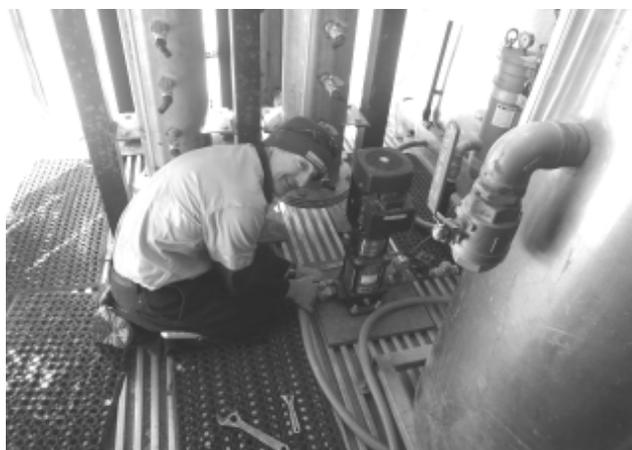
**Figure 4:** *Connecting up the pump pipework prior to commissioning*
