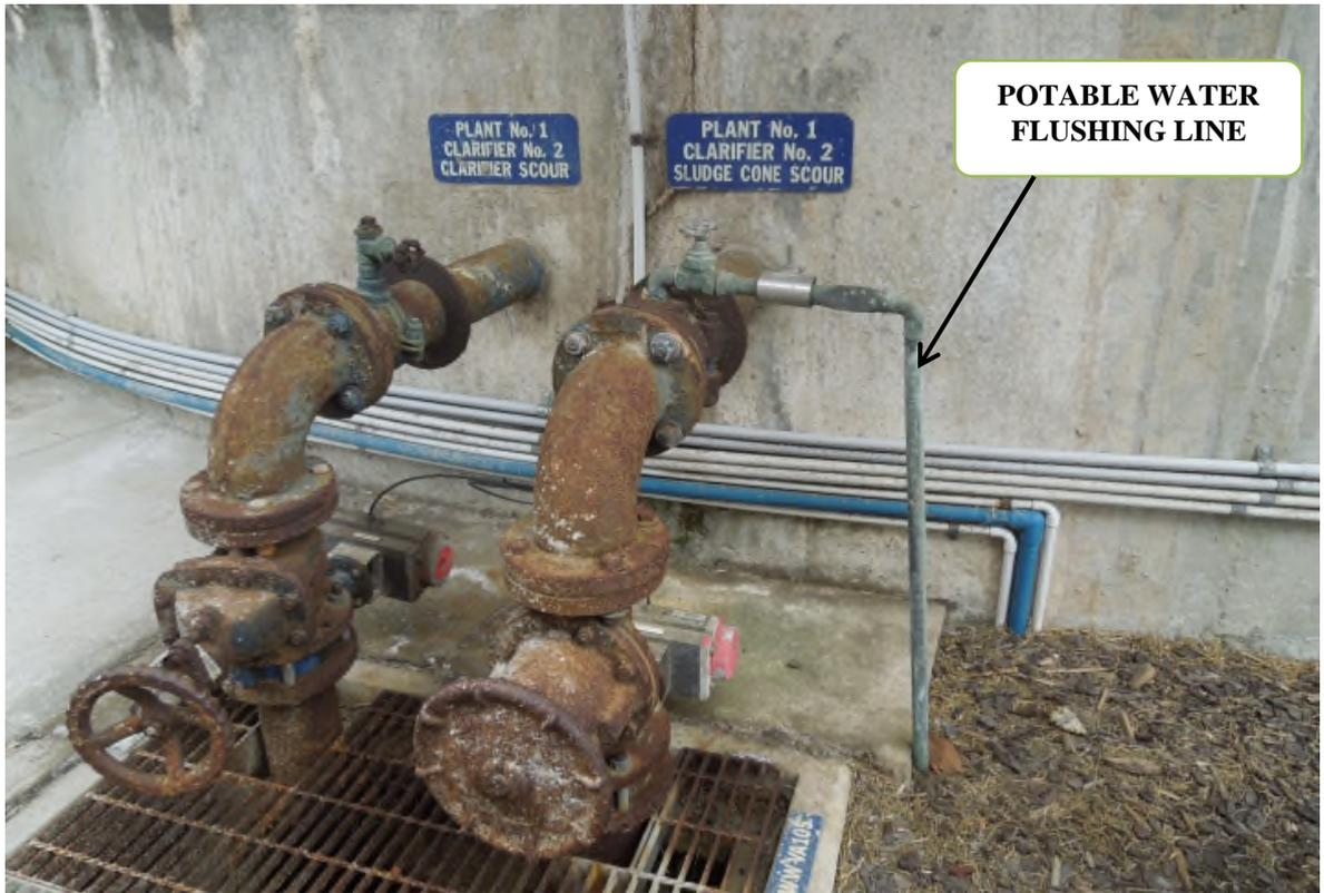
**Figure 2:** Clarifier de-sludge line cross connection
