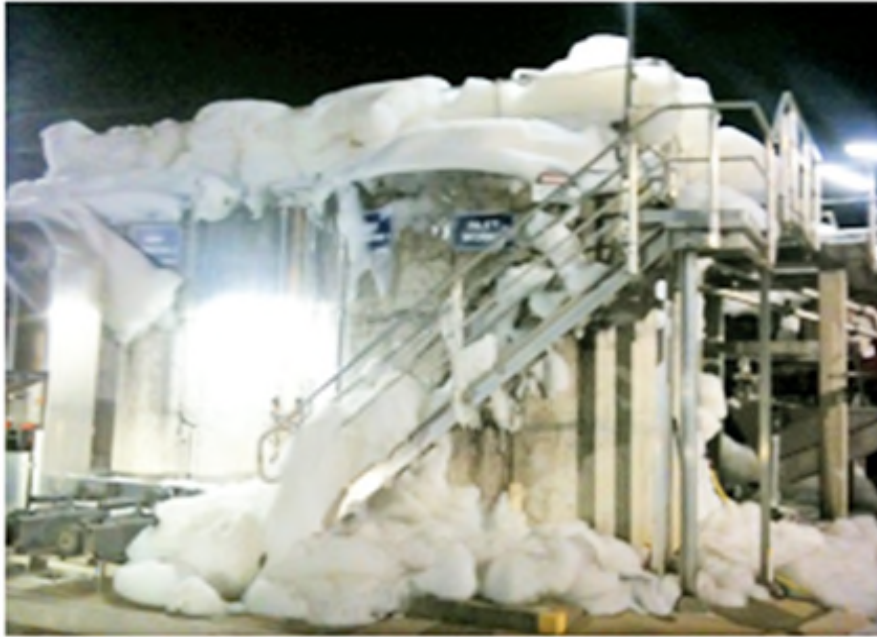
Figure 1: Trade Waste Shock at Inlet Works – Burpengary East STP.
