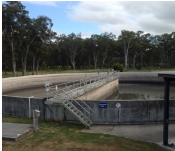
Figure 2: Four ML Raw Sewage Balance Tank (RSBT) – Burpengary East STP.
