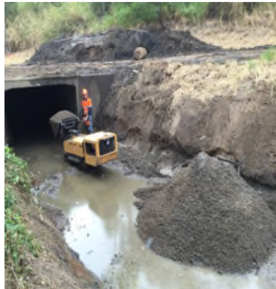
Figure 6: Microtraxx Hauling Back Debris.
