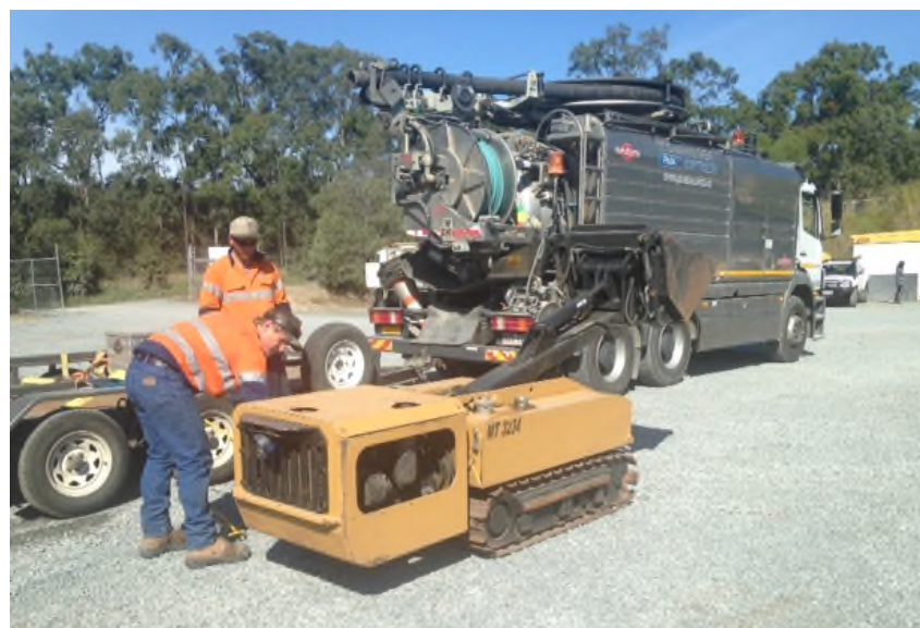
Figure 9: Equipment used on site Microtraxx and Drain cleaner/vacuum truck.
