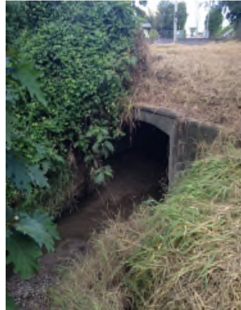
Figure 4: Headwall after Slashing.
