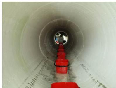
**Figure 6:** *MHL Coated Sewer Pipe*
