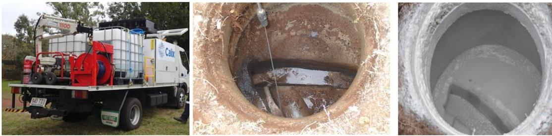
**Figure 7:** *Calix Coating Rig      Corroded Manhole      Ccoated Manhole*
