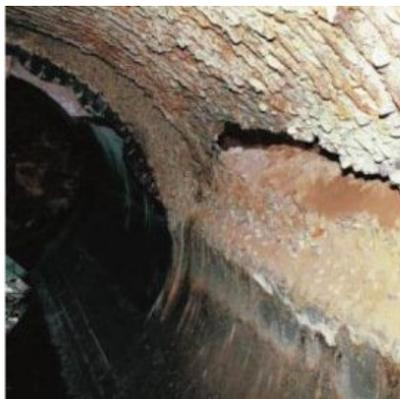
**Figure 2:** *Sewer Line Corroded by Acid Attack*
