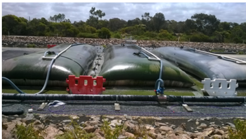
Figure 2: Geobags in Operation
