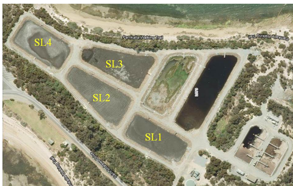
Figure 1: Port Lincoln WWTP: Overview
