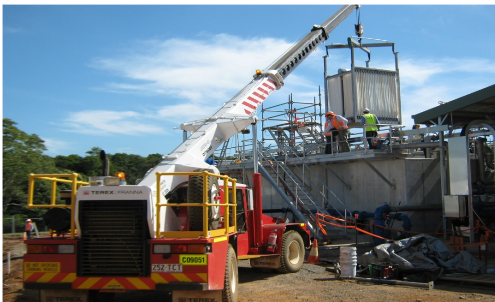
Figure 1: Construction Works Under Way
