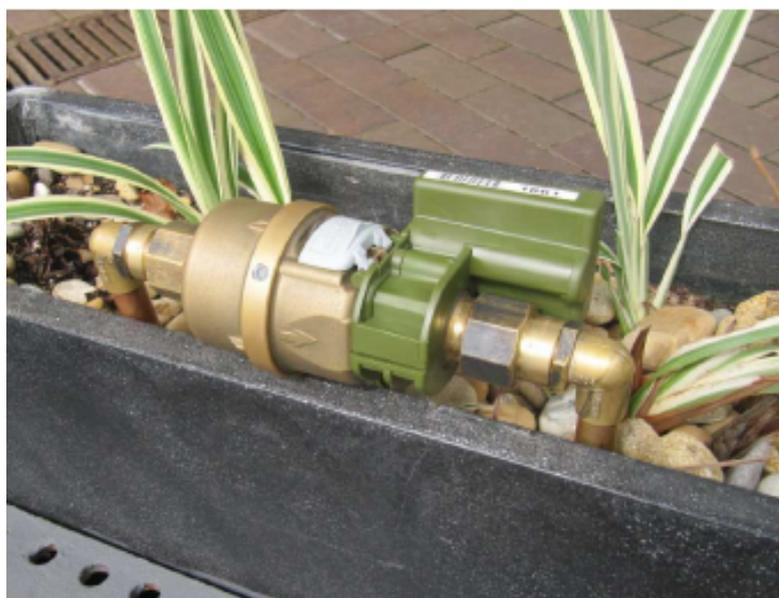
**Figure 3:** *Taggle Fitted Meter*
