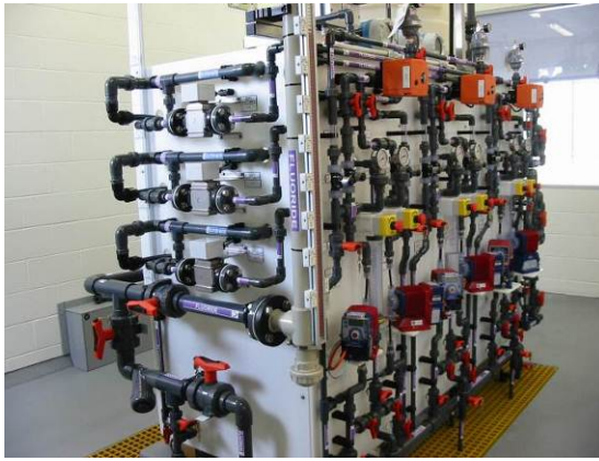
Figures 3 & 4: Fluoridation Dosing System at Rosewood Reservoir Site
