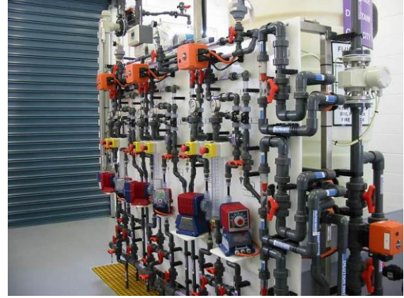
Figures 3 & 4: Fluoridation Dosing System at Rosewood Reservoir Site
