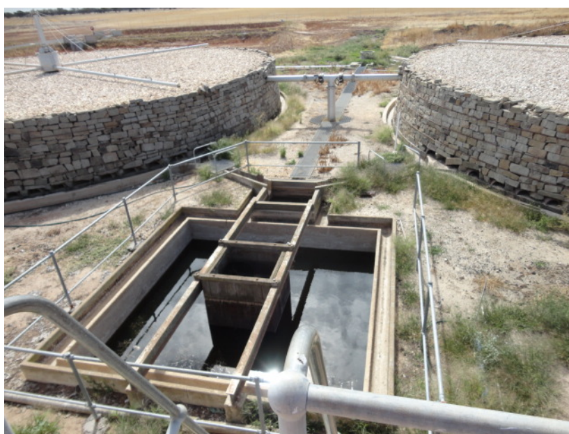
Figure 1: The original trickling filters at Warracknabeal WWTP
