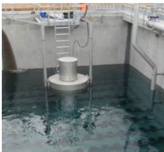
Figure 5: The linear decanter unit
