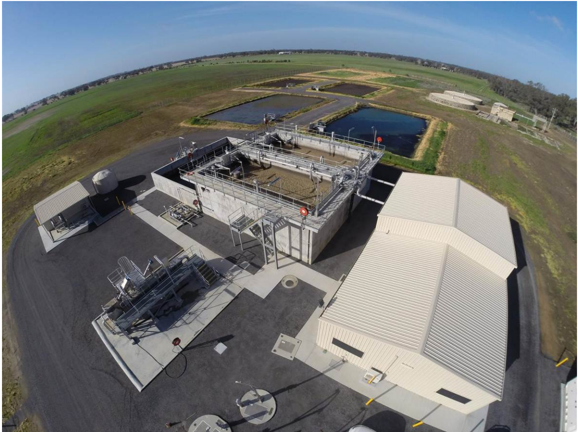
Figure 7: Aerial View of the new Warracknabeal WWTP
