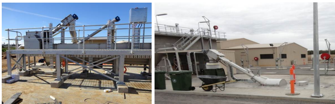
Figure 3: The inlet screens at Warracknabeal (left) and St Arnaud (right)
