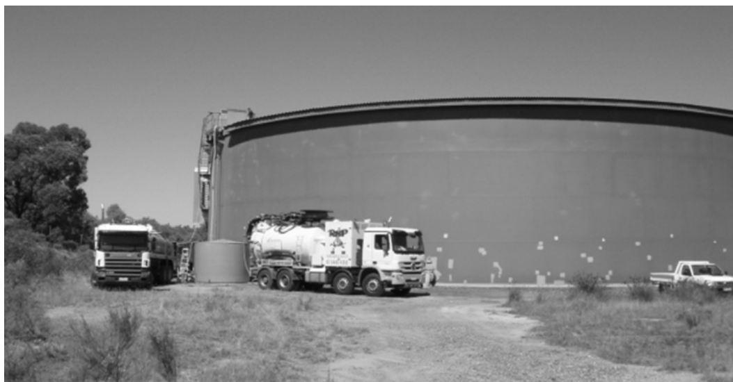
Figure 1: Edwards Road Tank, a 15ML storage on the Bendigo drinking water distribution network
