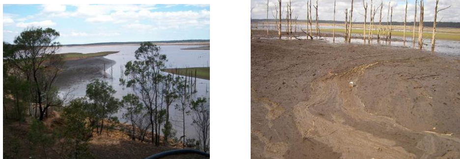
Figure 3: Coongulla raw water offtake buried in mud and debris.
