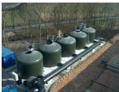
**Figure 3:** *Biotrickling filter*
