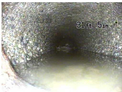
**Figure 5:** *Corroded concrete pipe*
