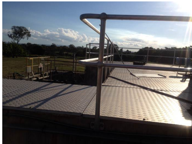
Figure 2: Inlet works with deteriorated walkways removed (left); after making the area safe (right)
