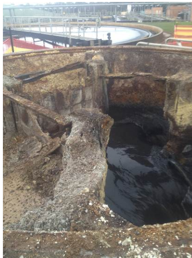
Figure 1: Existing primary clarifier flow splitter with covers removed
