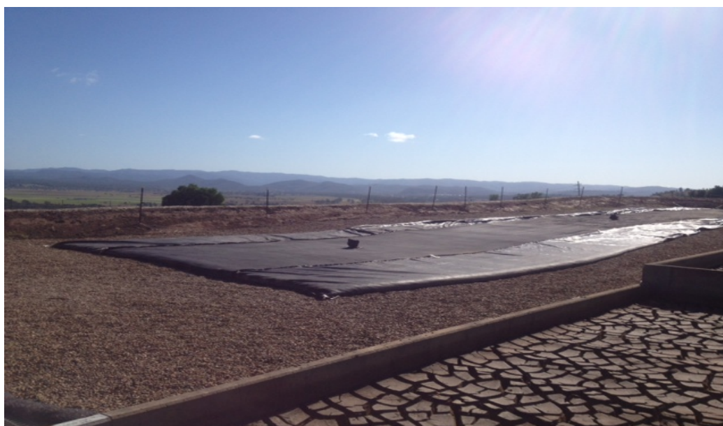
Figure 3: New geotube being commissioned
