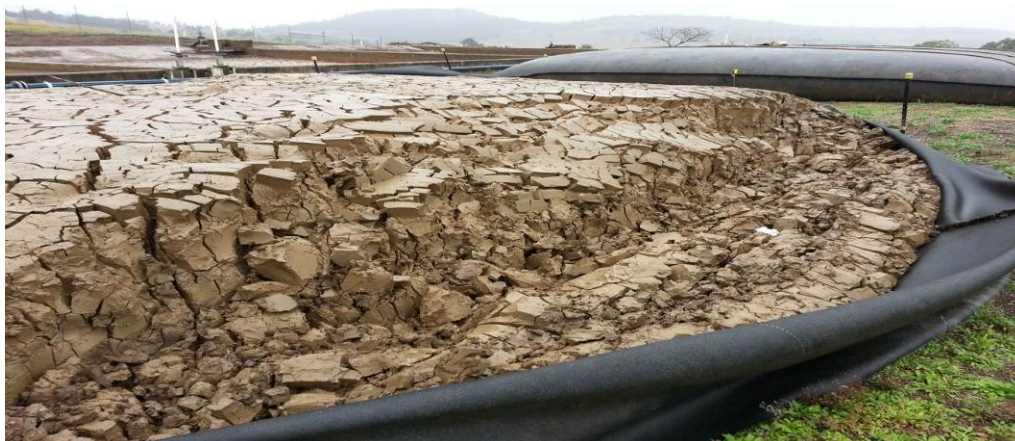
Figure 1: Photo showing geotube cut open for disposal
