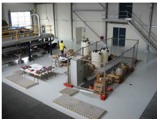
Figures 1 & 2: Wauchope WTP with the Fluoridation Dosing System Work Area & Final Dosing System Configuration
