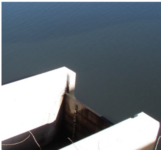
Figure 3: Old Drying Bed Decanting Weir Boards
