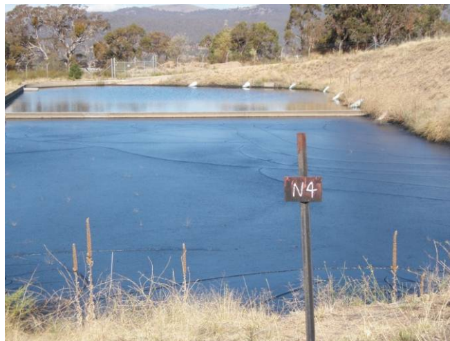
Figure 1: GWTP drying beds North 4 (foreground) and South 4 full of PAC sludge.
