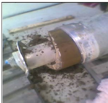
Figure 4: Blocked centrifuge that led to significant period of down-time for the Woodglen WTP washwater system.
