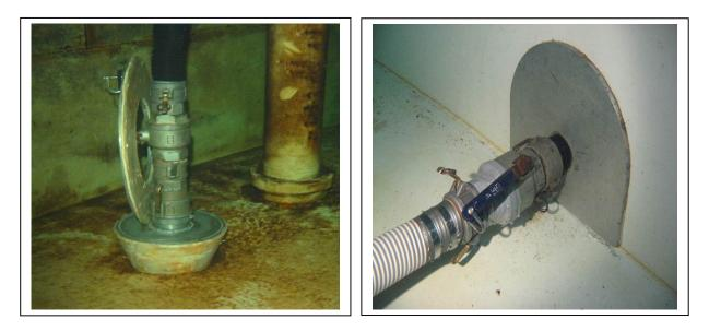
On elevated tanks, and having no scour access, a siphon can be created. This is preferable to hanging hard hoses long distances down to a pump for priming. The more heavy hose lowered over the side of a high tank, the greater the chance of a connection failing and causing an incident to the personnel working below. Lighter weight lay-flat hose can be used below the siphon point to run the waste water away.
