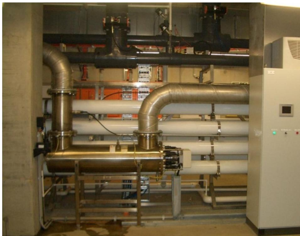
**Figure 3:** *Ultrafiltration and UV disinfection units*
