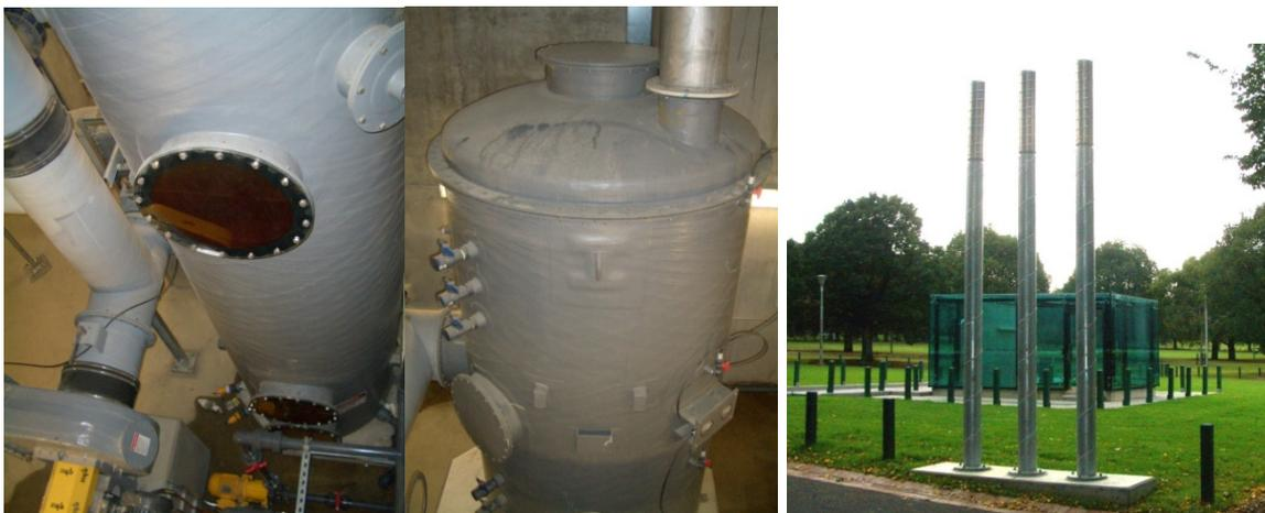
**Figure 4:** *Odour Control Unit (OCU) chemical scrubber tower, Carbon Filter vessel and surface ventilation stacks*
