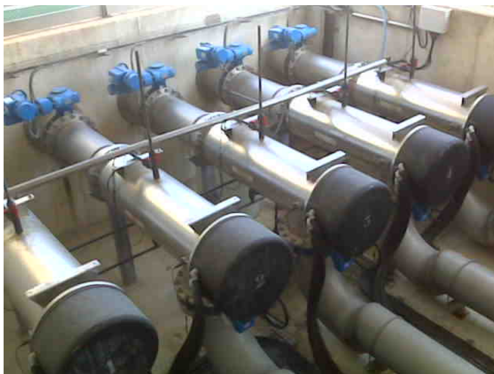
Figure 1: Five 32AL50 UVFit™ closed vessel reactors installed in parallel in Spain for disinfection of filtered secondary effluent. The reuse water was used for an irrigation application.
