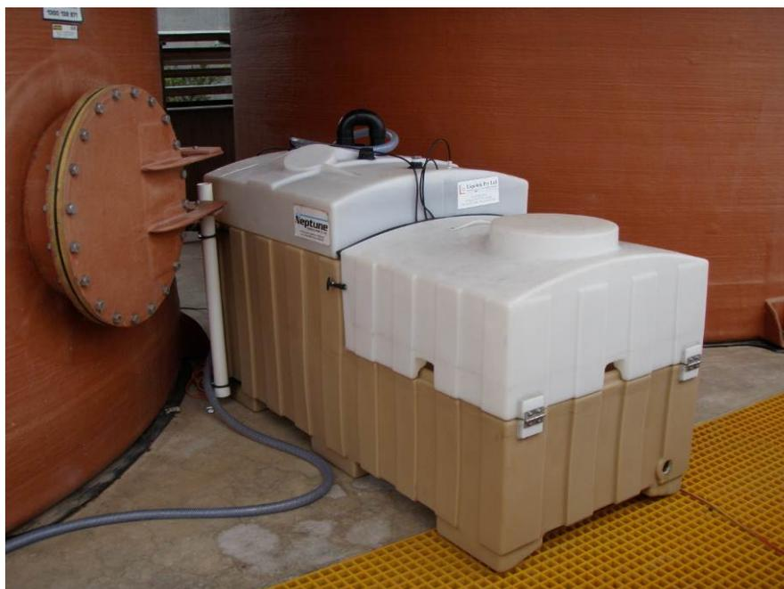
**Figure 3:** Alum dosing skid
