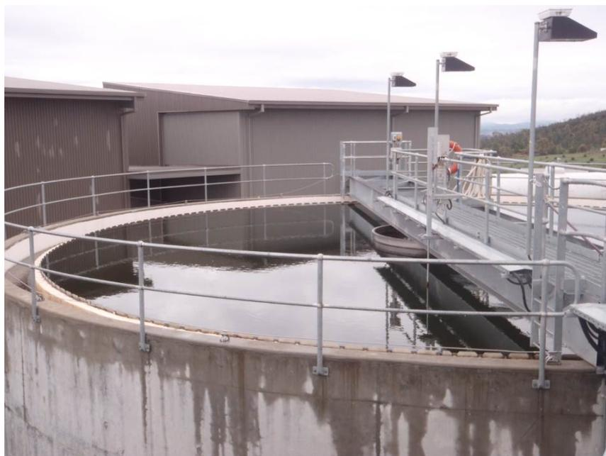
**Figure 2:** *Sludge Thickener*
