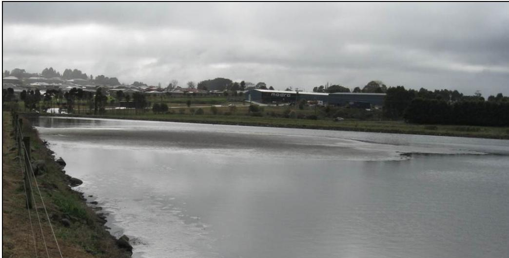
**Figure 1:** *WWTP settlement lagoon showing zone of sludge buildup at surface*
