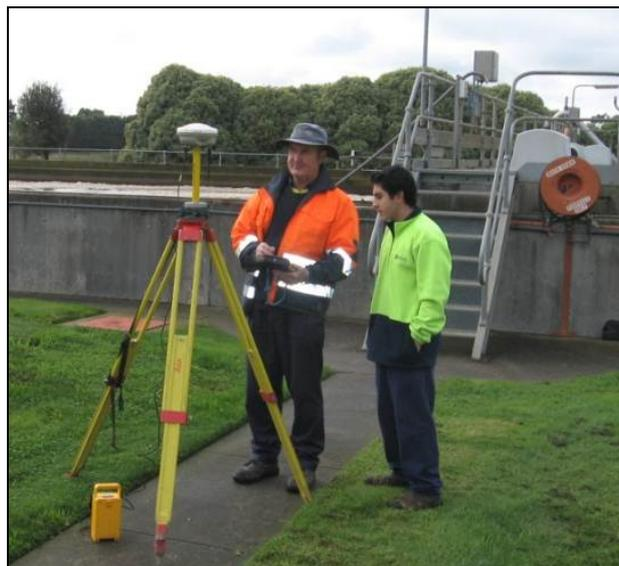
**Figure 2:** *Establishing Survey Base Station Prior to Survey Commencement*
