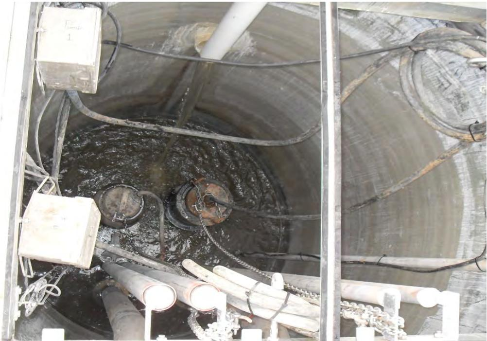
**Figure 2:** *Merrijig Sewage Pump Station – New fiberglass tank*
