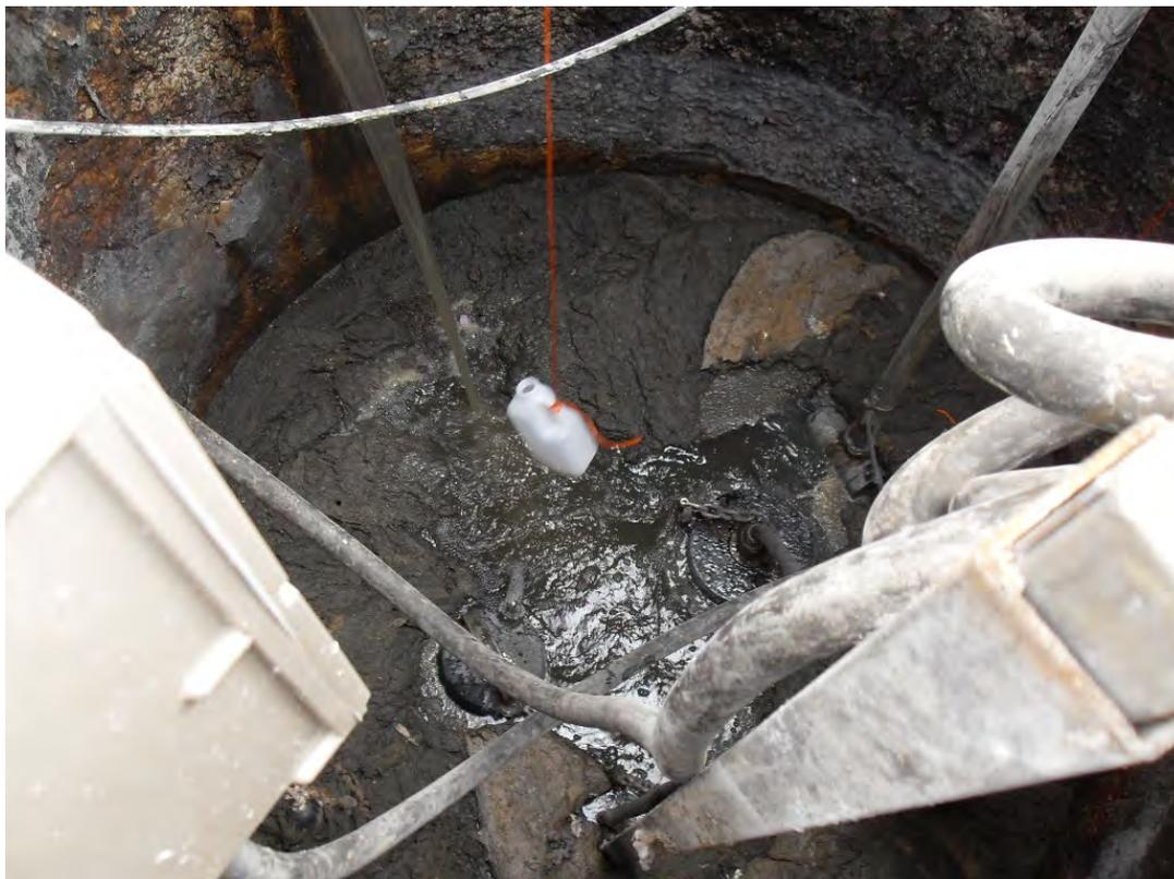
**Figure 1:** *Merrijig Sewage Pump Station – Note side walls of Wet Well*
