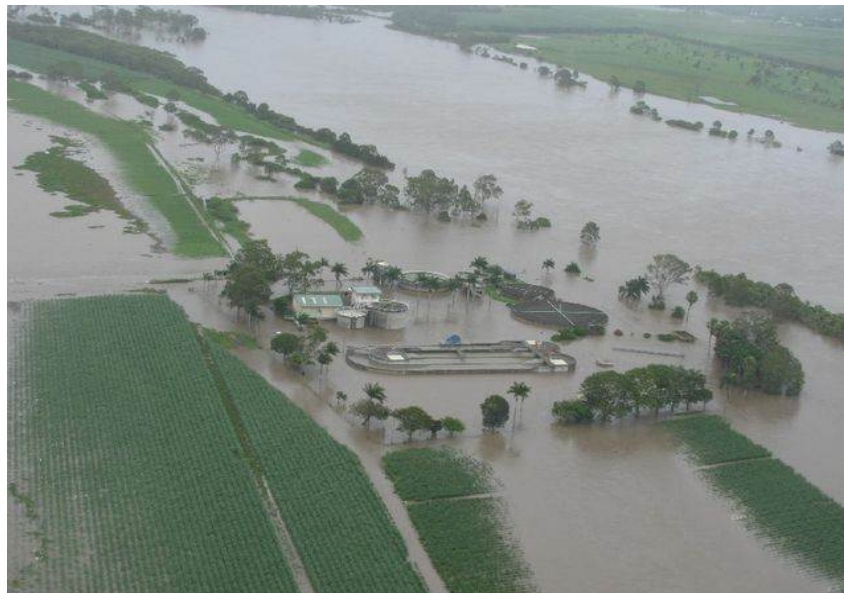
Figure 3: Millbank WWTP at Flood Peak
