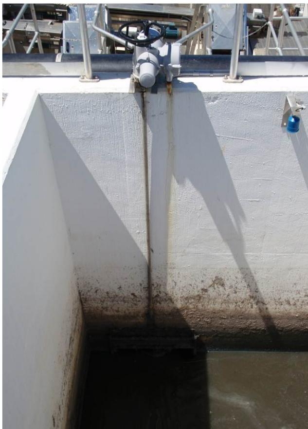
**Figure 2:** *Rotork operated penstock on outlet of balance tank*
