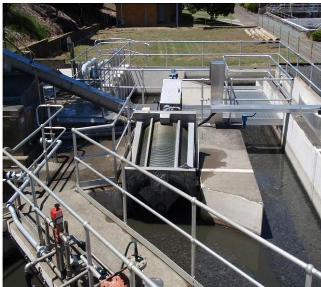
**Figure 1:** *Drum screen installed post grit arrestor.*
