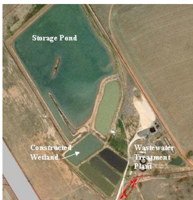
Figure 1: Junee Wastewater Treatment Plant
