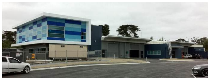
Figure 1: National Water Resource Training Facility at Chisholm's Water Center
