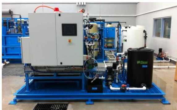
Figure 7: Submerged Ultra-filtration module
