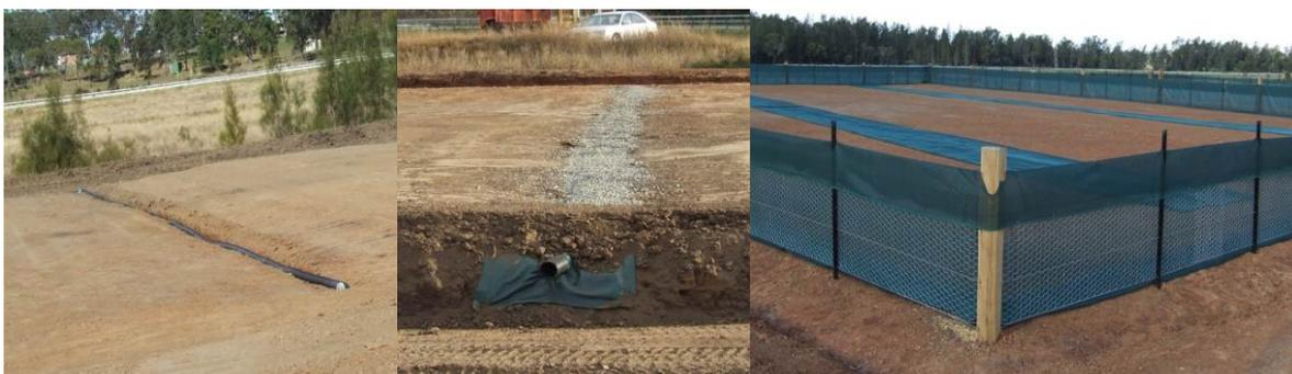
**Figure 1:** *Ground compaction, agricultural pipe installation and ready to use bed*
