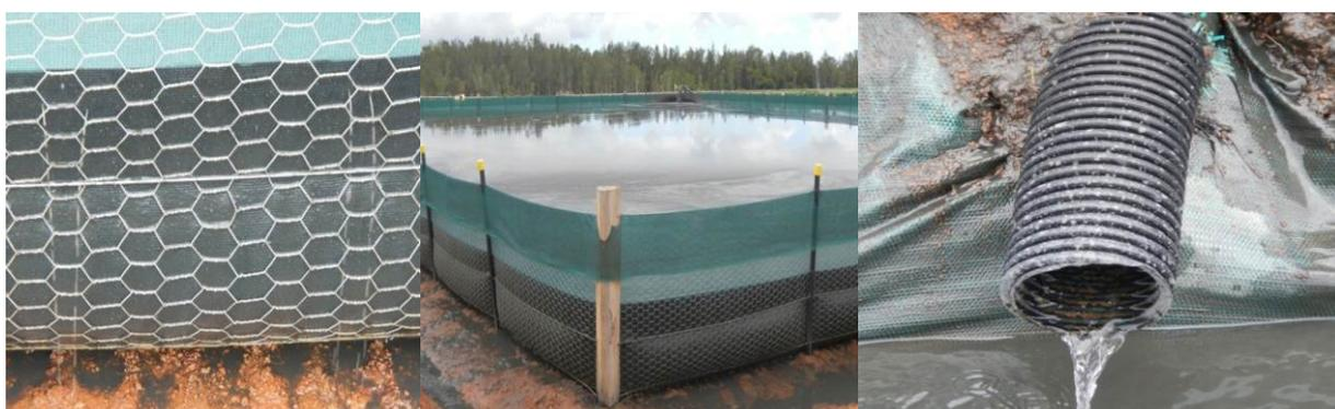
**Figure 2:** *A close ups-the filtrate through fencing, a full bed and supernatant via under bed drainage*
