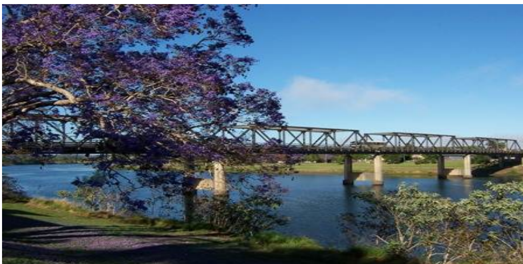
Figure 1: Pacific Highway Bridge at Kempsey
