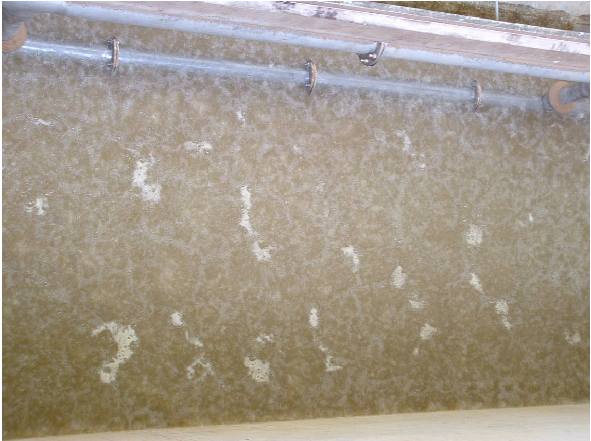
Figure 5: Resulting air scour pattern from new system.
