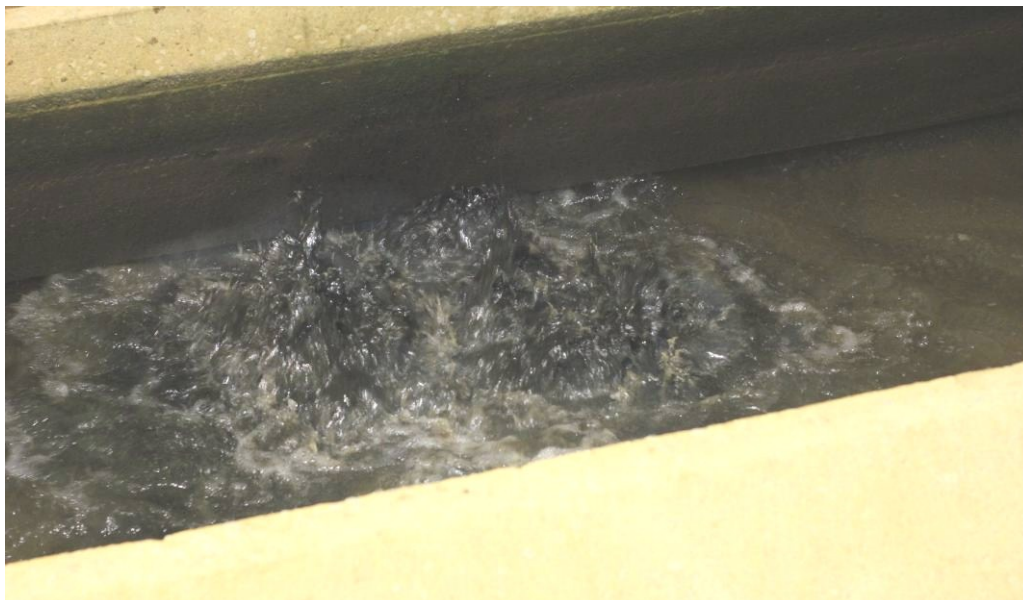
Figure 1: Eruption at the start of an air scour sequence
