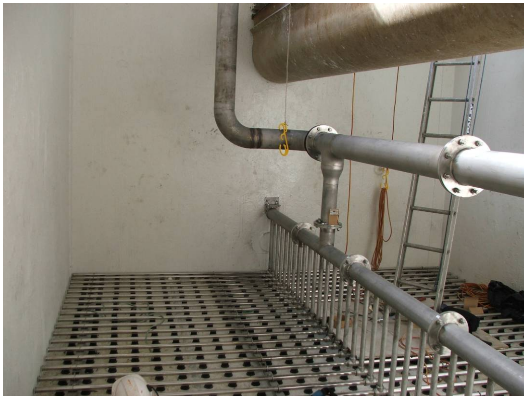
Figure 3: Arrays in flanged sections for easy installation.
