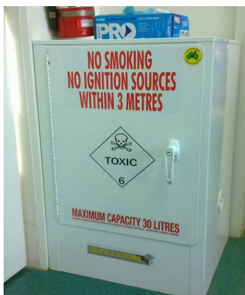
Figure 2: Storage vessel and containment for manganese reagent and waste
