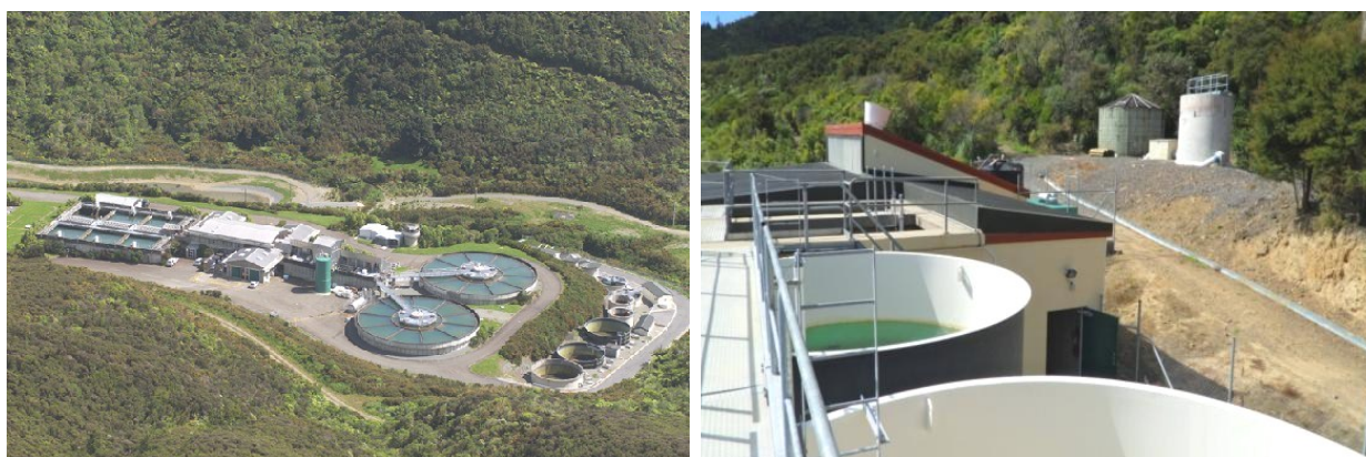
Figure 2: Te Marua WTP and Te Aroha WTP
