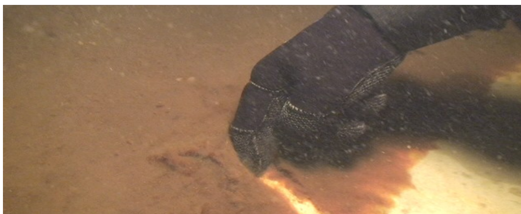
Figure 2: Sludge layer in clear water storage
