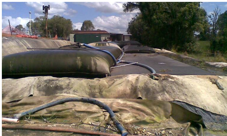
Figure 2: Geotextile bags configuration
