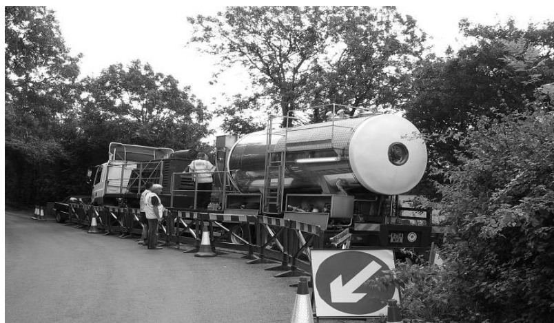
Figure 2: The ice delivery truck onsite ready to begin pigging
