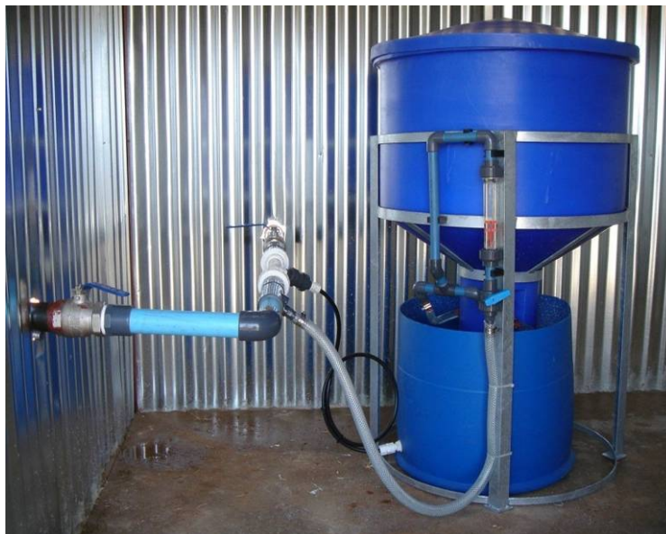
Figure 6: Feeder with reservoir using a partial vacuum or venturi system to draw the CH solution from the reservoir below the feeder into the main water supply.
