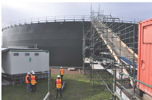
Figure 6: Scaffold ready for Kalzip installation
