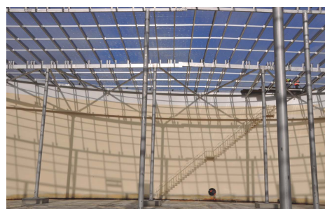
Figure 5: New stainless steel roof subsystem and safety mesh
