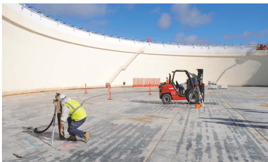
Figure 2: Cementitious grout injection
