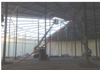
Figure 4: Deconstruction of the roof
