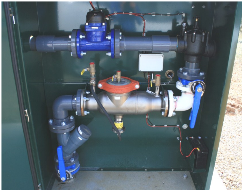
Figure 2: Pipe work arrangement of water filling station
