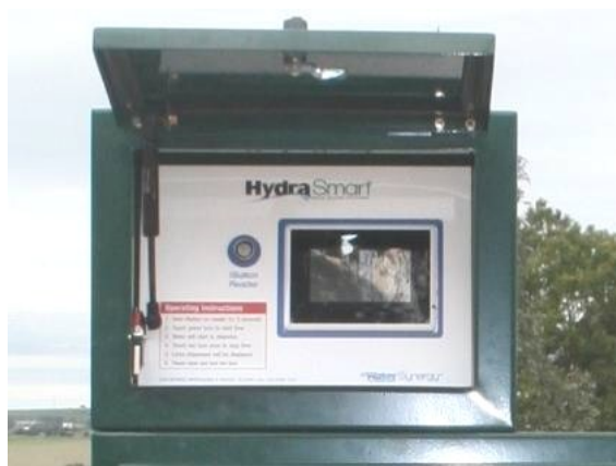
Figure 3: Touch screen interface and iButton scanner
