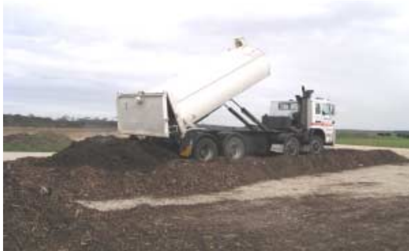
Figure 1: Biosolids being deposited upon a bed of green waste.
