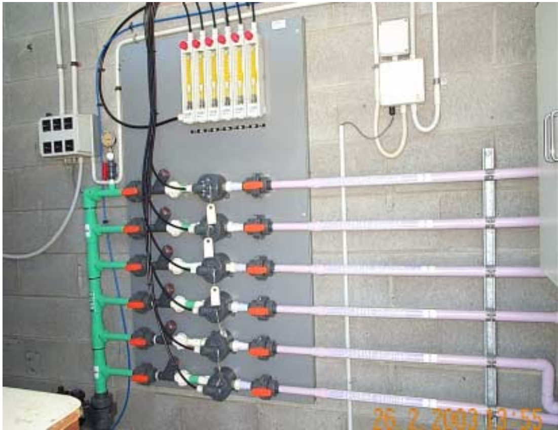
Figure 4: Chlorine Injection Network
