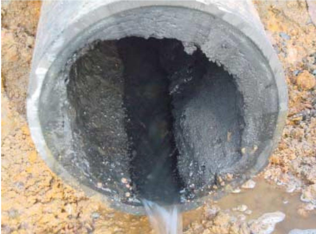
**Figure 2:** *Sludge Build-up in Sewer*
