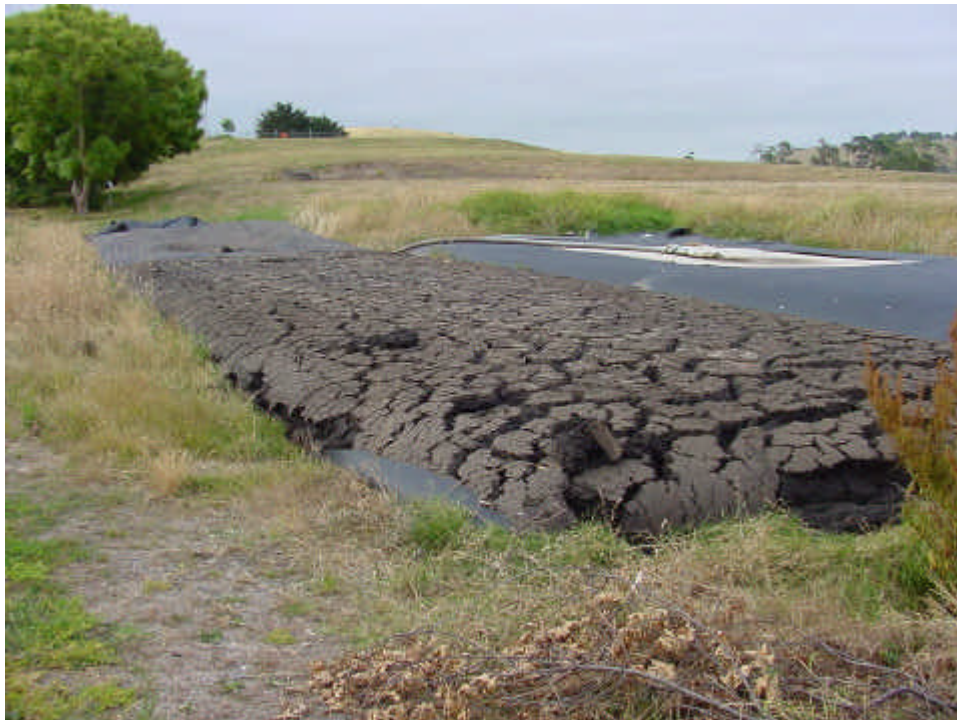
Figure 1: Initial bag at Korumburra approximately two weeks after opening with second bag still filling in background
