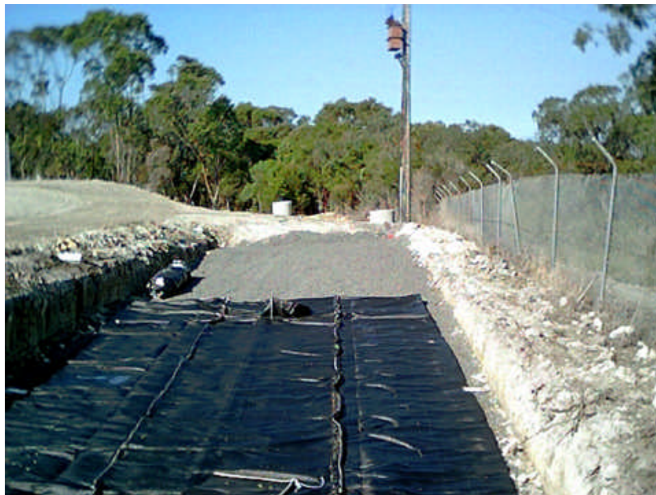
Figure 5: Prepared bed at Foster WTP with first Geobag in place
