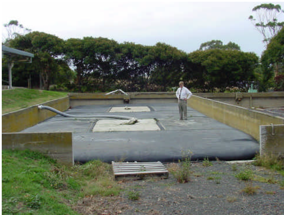
Figure 2: Leongatha Geobag after approximately six months of use
