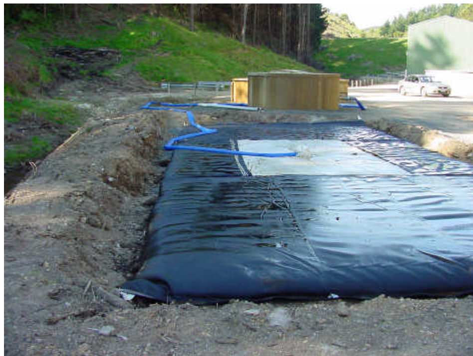
Figure 4: Fish Creek Bag during initial filling Sludge holding tank in background
