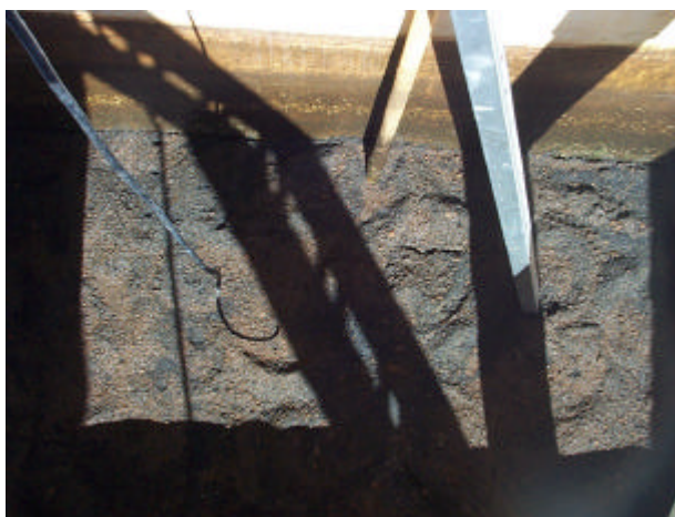
Figure 2: Uneven media surface, as a result of the filter inlet design
