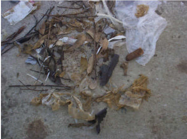
Figure 6: Rubbish removed from within the filter during refurbishment at Sale
