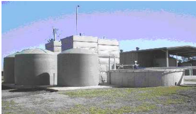
Figure 1 - Heyfield Water Treatment Plant
