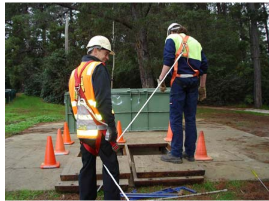
Figure 5: Fall restraint lines can become tangled and potentially create additional hazards.
