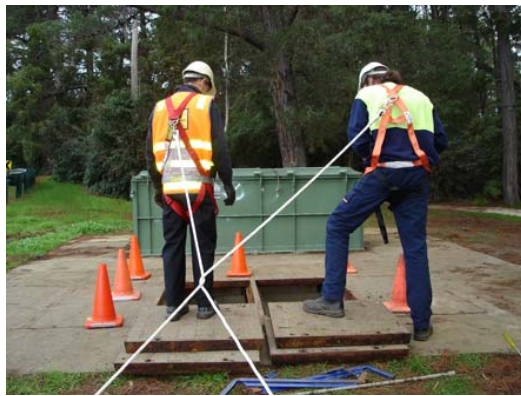
Figure 5: Fall restraint lines can become tangled and potentially create additional hazards.
