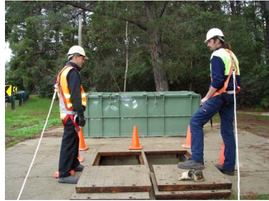
Figure 4: Gatic lids open, persons tethered to anchor points.
