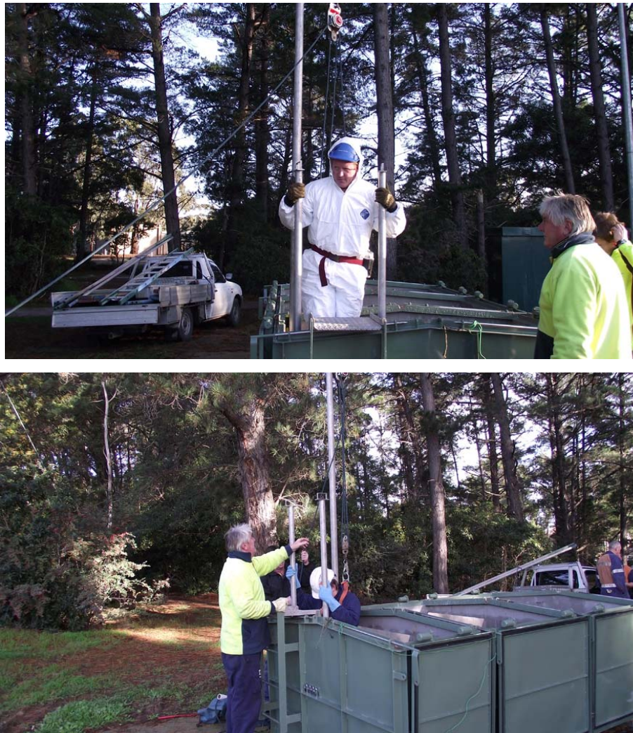
Figure 8: Workers accessing the wet well using the ladder and davit arm.
