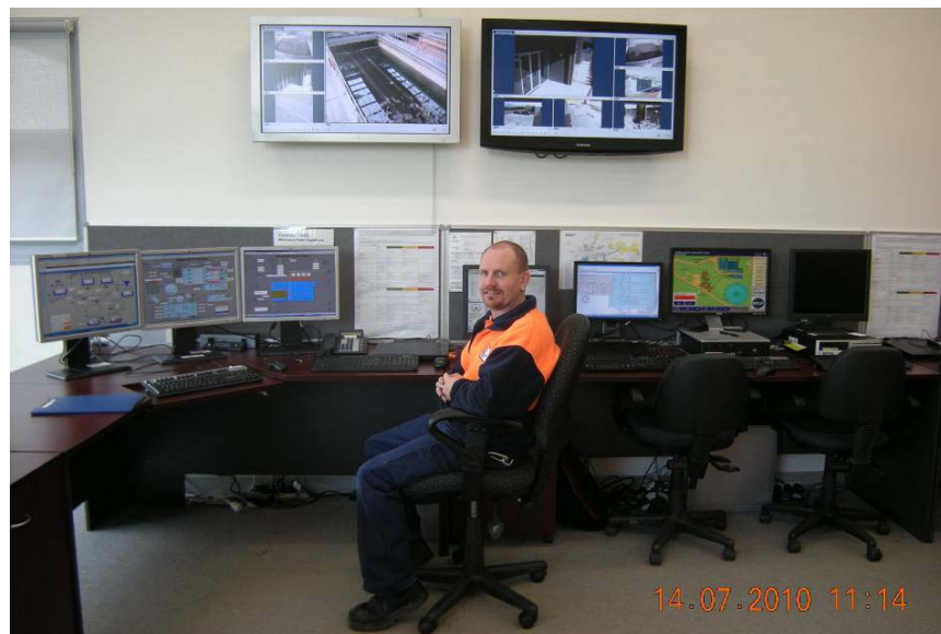
Figure 2: Lead Operator Gary Anderson in the Tarago WTP Control Room
